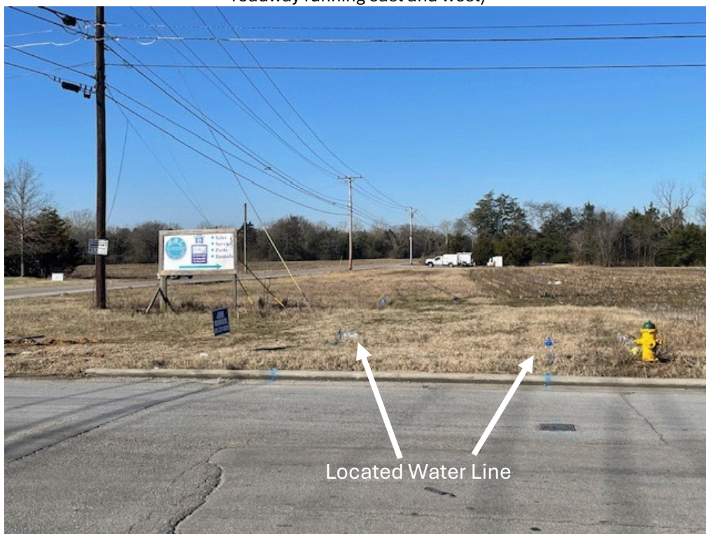
Power and Water Lines – Intersection of Capital Way and Epps Mill Rd facing west
