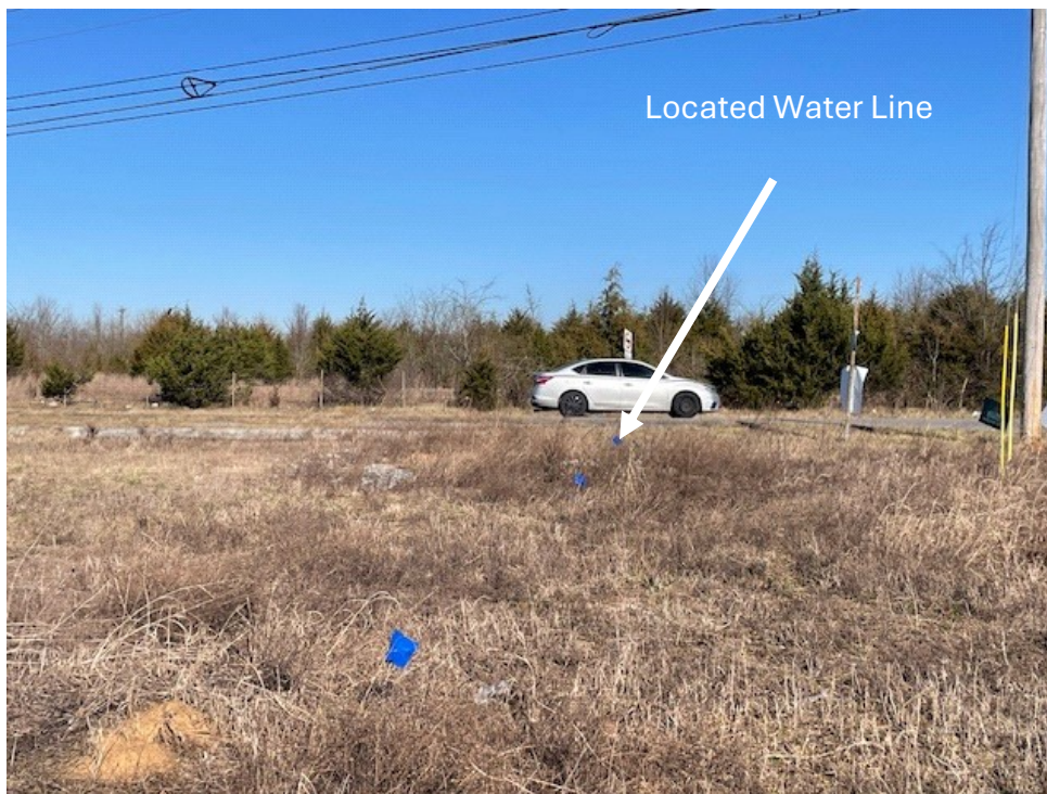
Water Line – Intersection of Miller Rd and Epps Mill Rd facing north (water line runs under Epps Mill Rd to north side)
