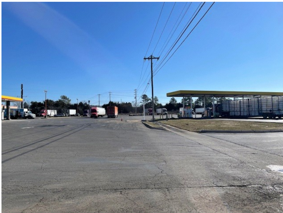
Power Lines – Shell station off Miller Rd facing east (power lines crossing interstate)
