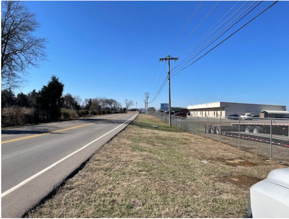
Power and AT&T Cable – Epps Mill Rd facing west between Manchester Pike and I-24
