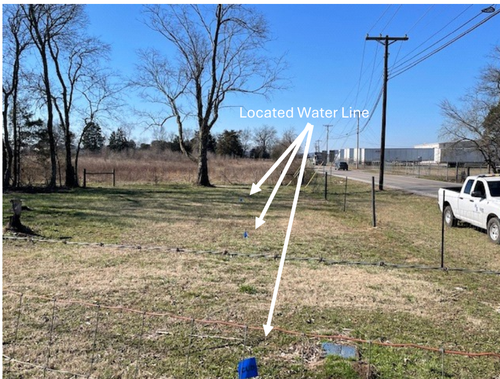
Power and Water Lines –Epps Mill Rd at Manchester Pike intersection facing southwest
