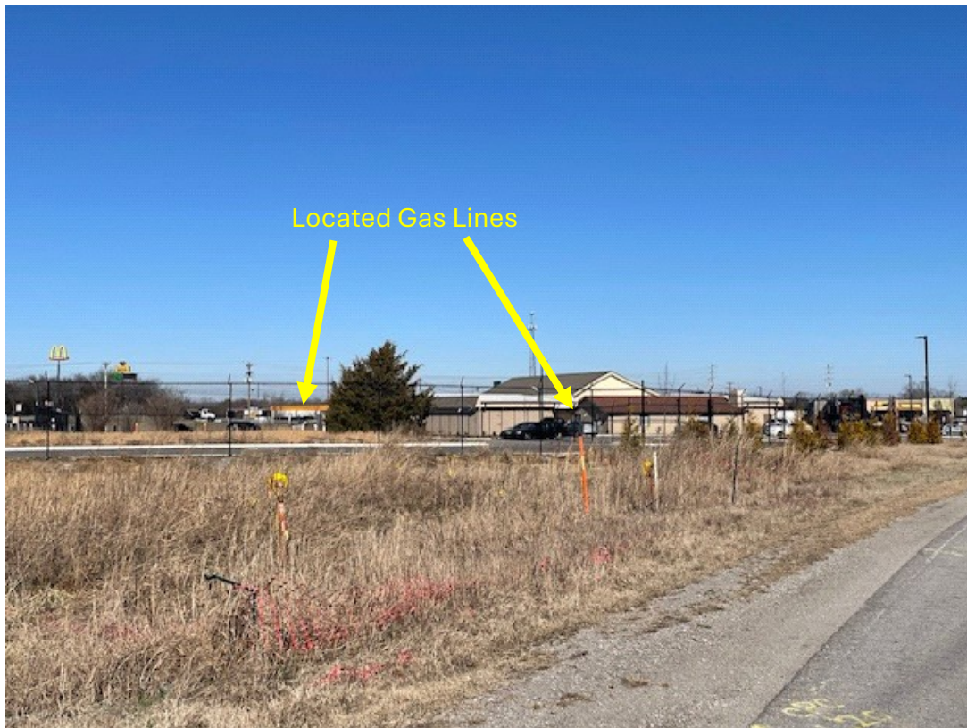
Gas Lines – Forbus Dr facing northwest
