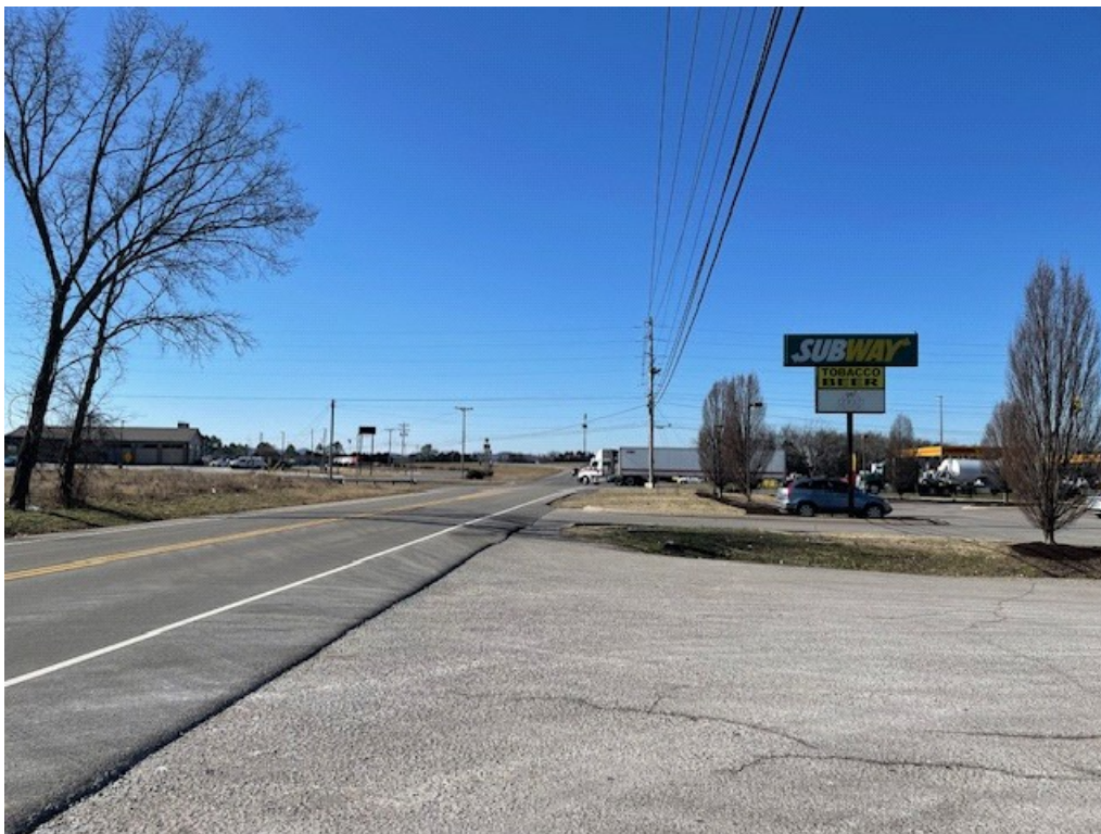
Power and AT&T Cable – Epps Mill Rd near Forbus Dr intersection facing southwest
