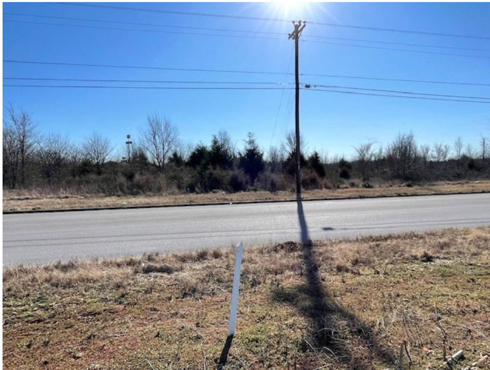
Power and Water lines – Capital Way facing east (3 rd pole from intersection, water line crosses under roadway running east and west)
