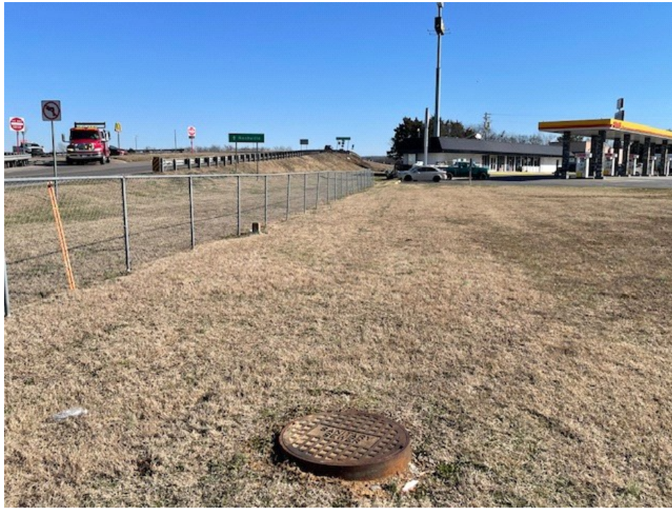
Sewer Manhole – Intersection of Miller Rd and Epps Mill Rd facing east
