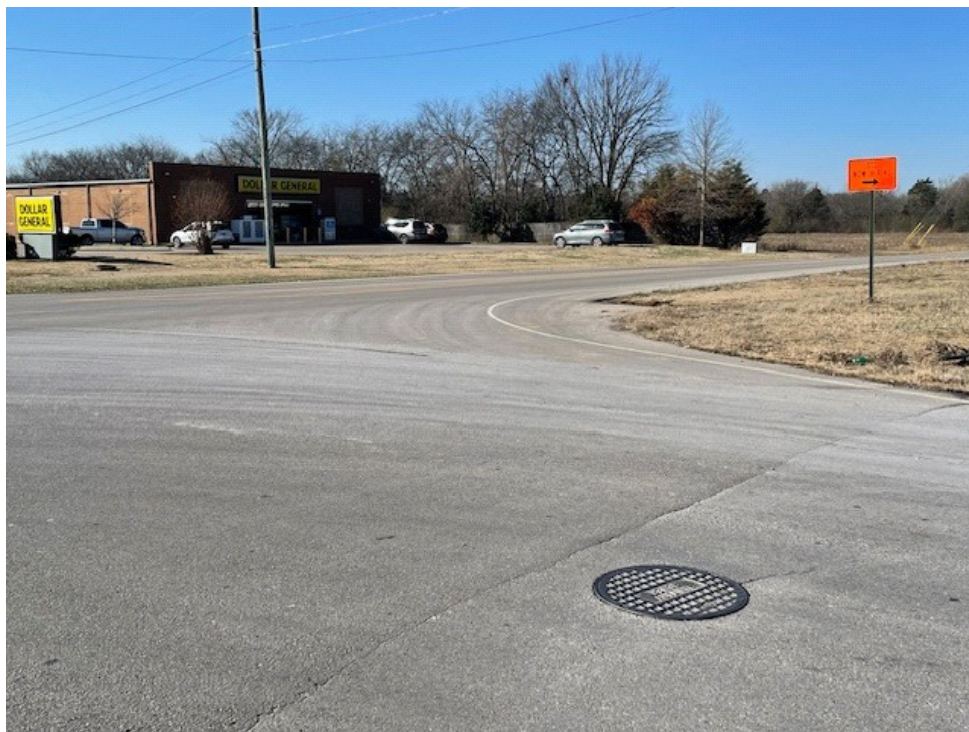
Sewer Manhole – Intersection of Capital Way and Epps Mill Rd facing southwest
