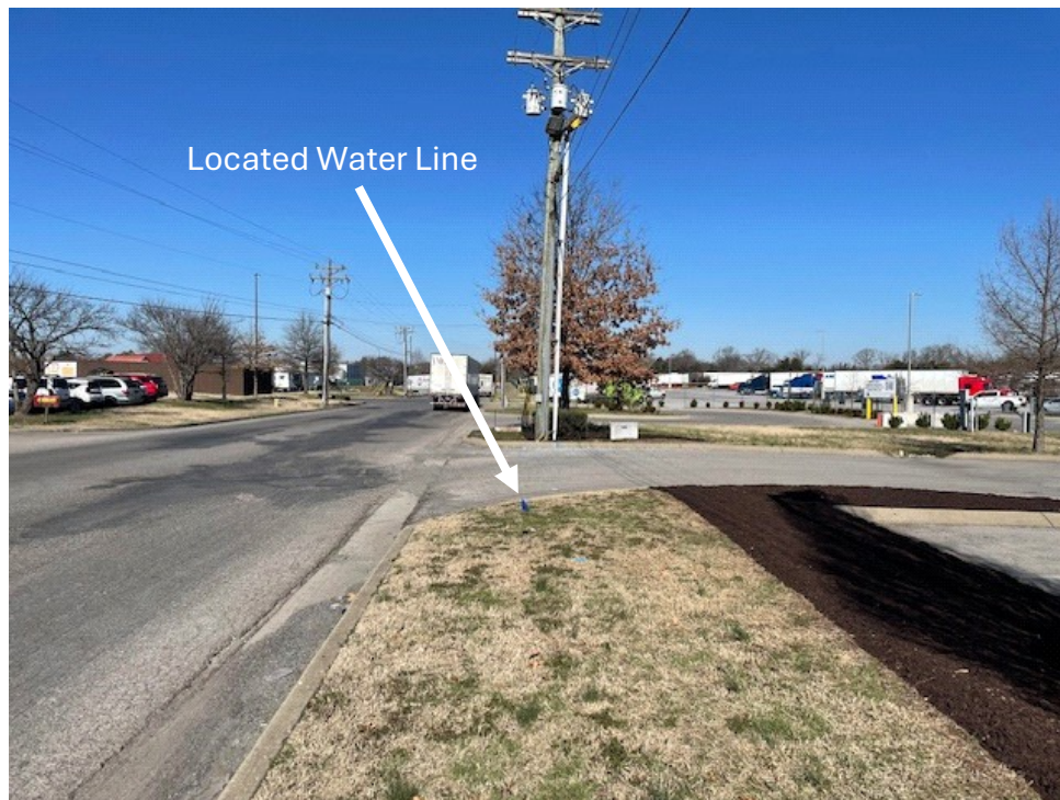
Power, AT&T, Water Lines – Forbus Dr (north side) facing northwest
