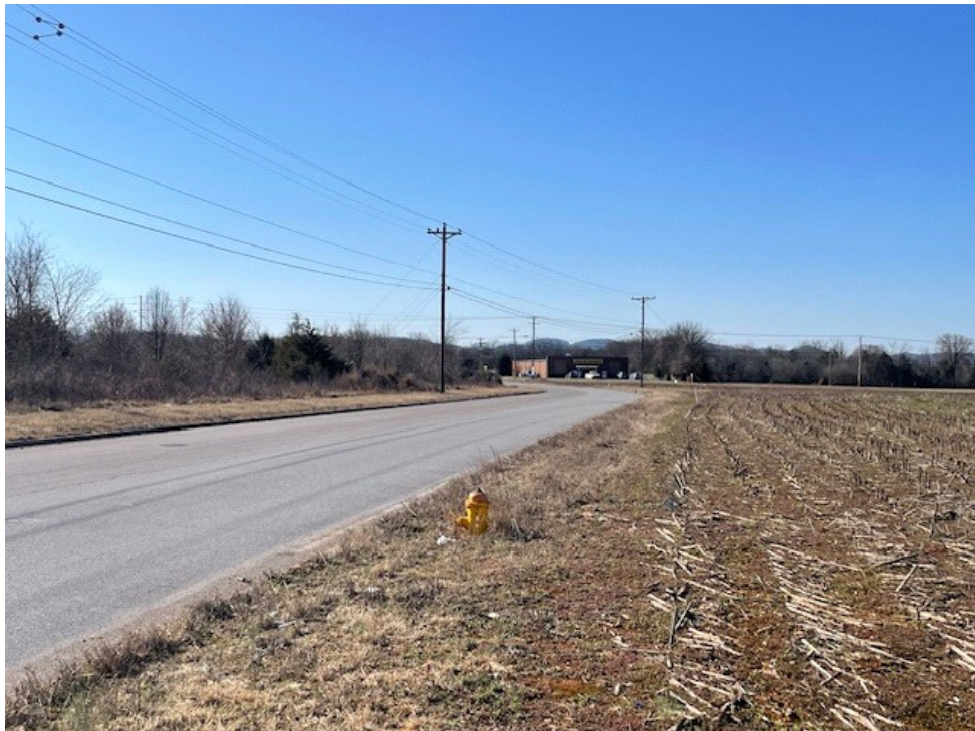
Power Lines & Hydrant – Capital Way facing south
