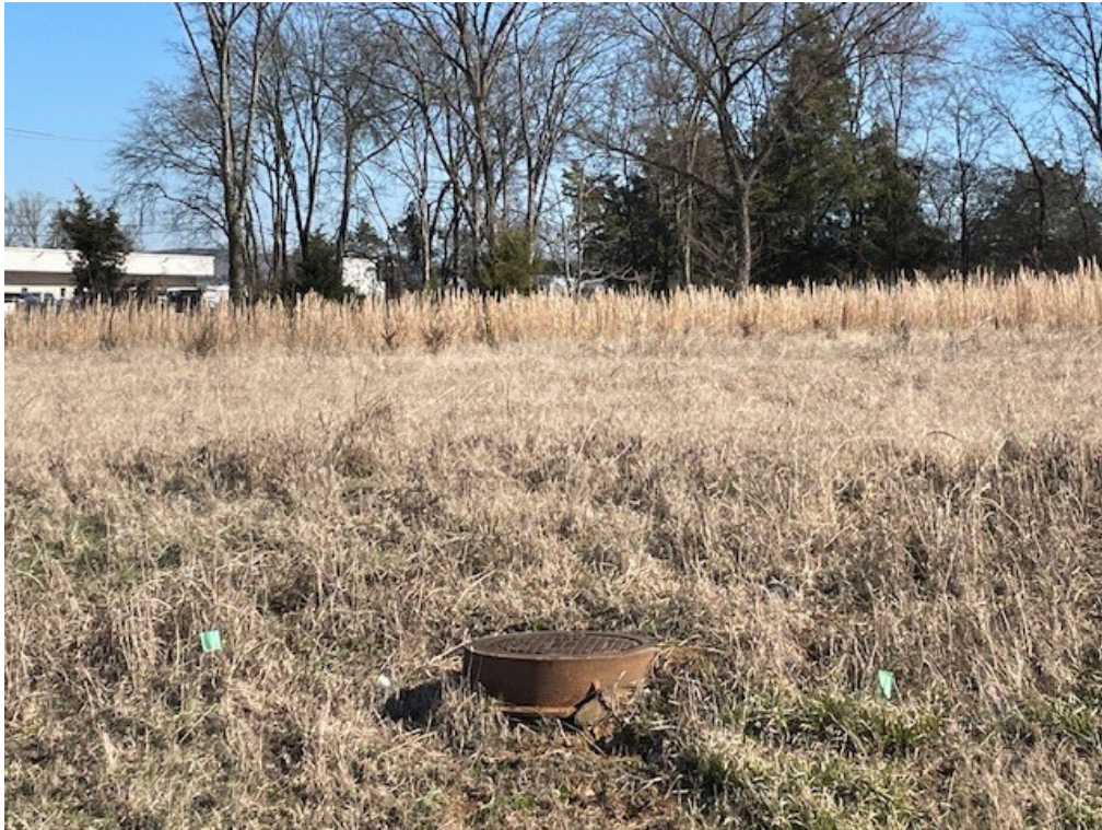
Sewer Manhole– Intersection on Forbus Dr and Epps Mill Rd east
